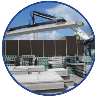
Concrete Floor Handling
