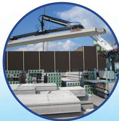
Concrete Floor Handling
